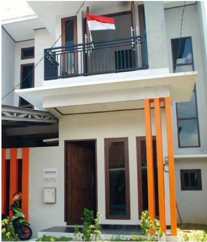
The new HOSCH building in Indonesia: offices and warehouse on the ground floor, living quarters on the second floor.
