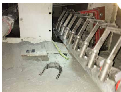
The D2 scraper in operation at a quarry owned by Norsk Stein A/S.
