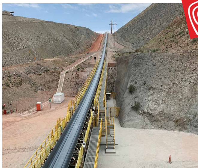
A technician is to be permanently deployed to service the conveyor belts of the Peruvian copper industry.
