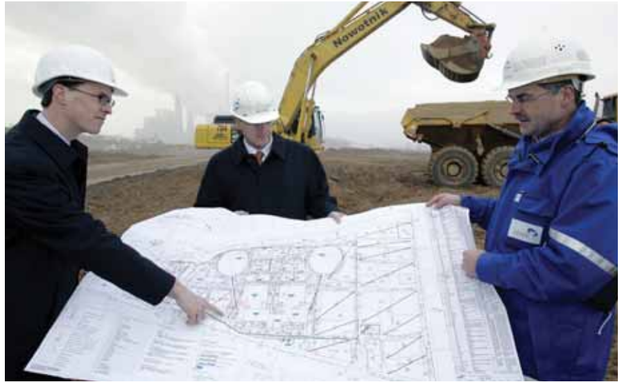
A new power station is being built in Neurath (Lower Rhine) – HOSCH takes part.
