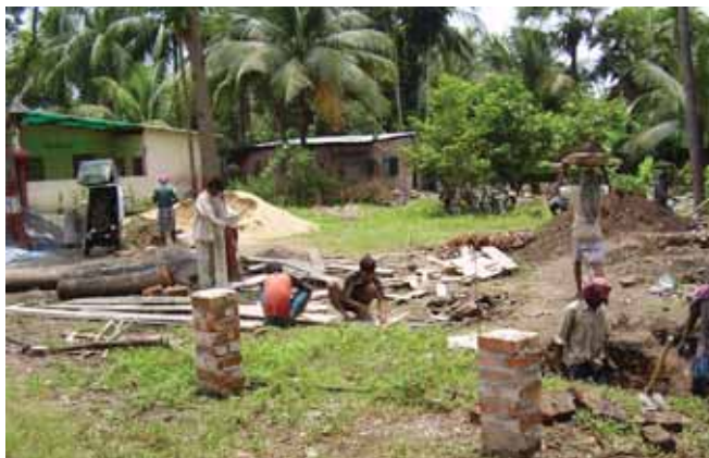
Construction on the site in Calcutta has already begun.
