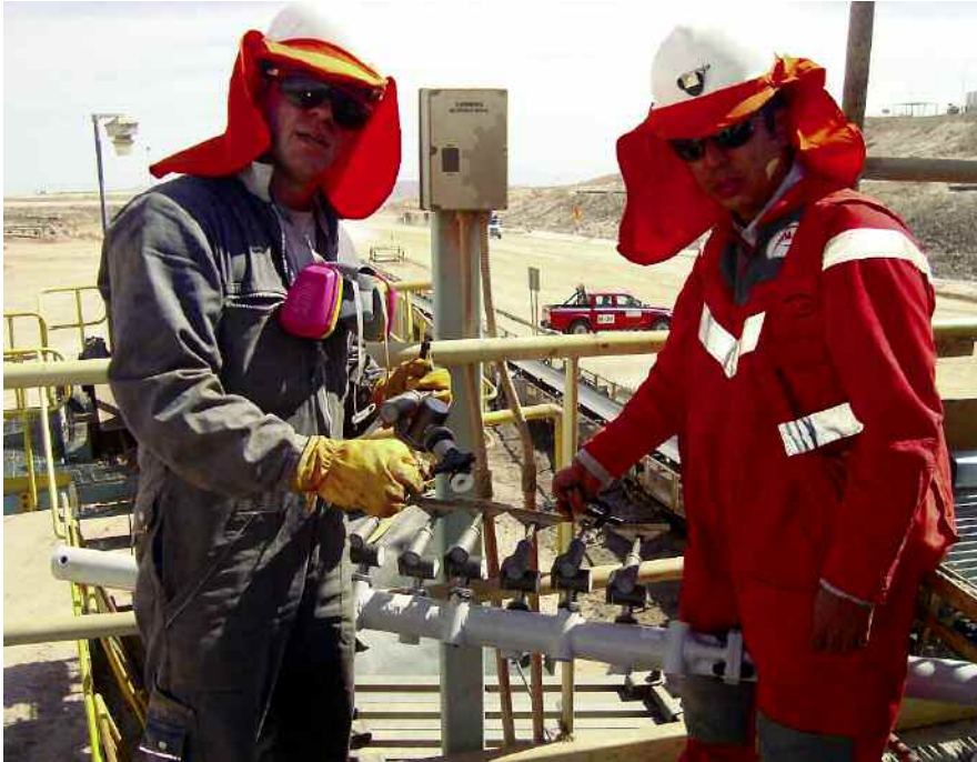
Heat and high altitude: the grueling conditions during the installation work in Chile ...
