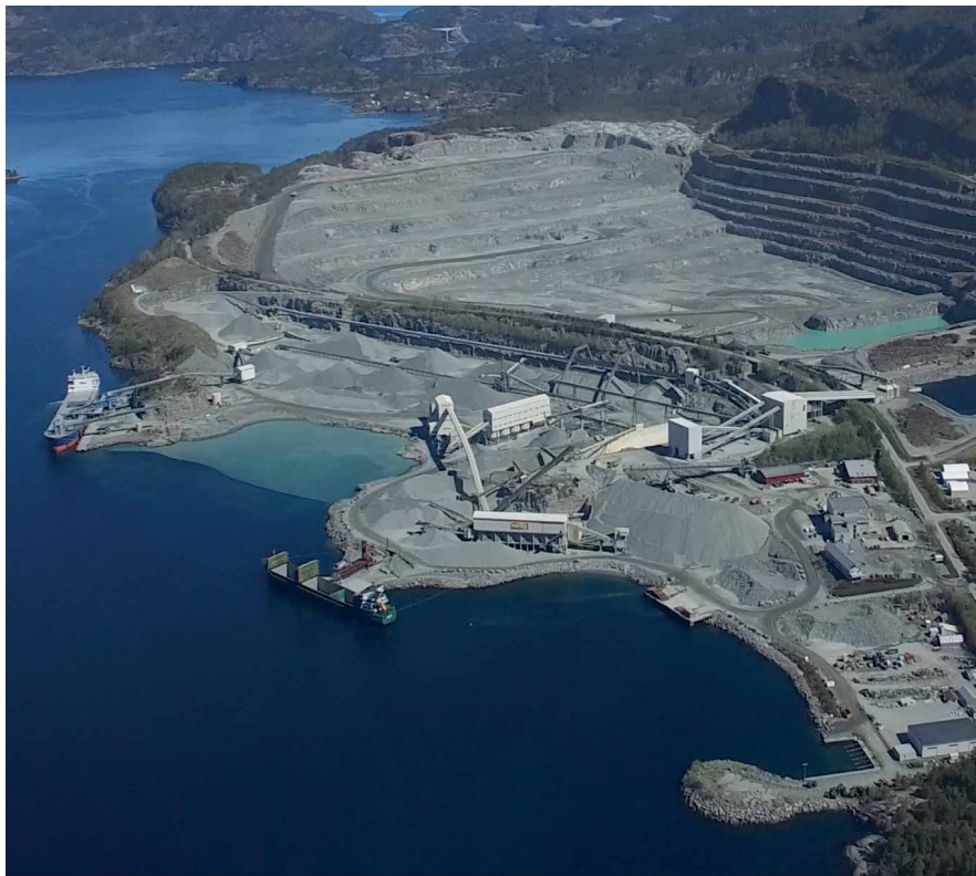
The Norsk Stein A/S facility on the Jelsa fjord near Stavanger is the largest quarry in Europe.
