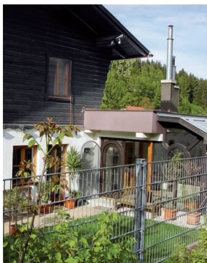
The HOSCH Austria office moves into this house in Techelsberg, very close to Poertschach on the Woerthersee
