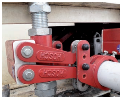
The special scraper in operation
