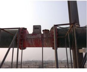
PSI at cyclone overflow in a bauxite processing plant
