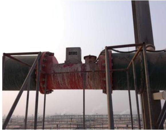
PSI at cyclone overflow in a bauxite processing plant
