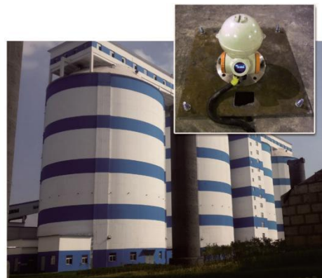
Clean coal silo at coal washery
