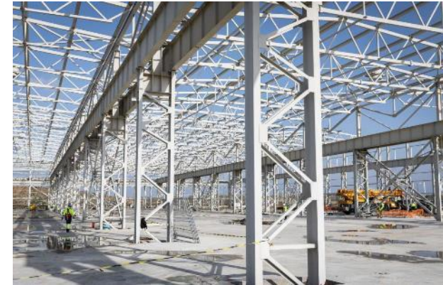
Rebar assembly workshop
