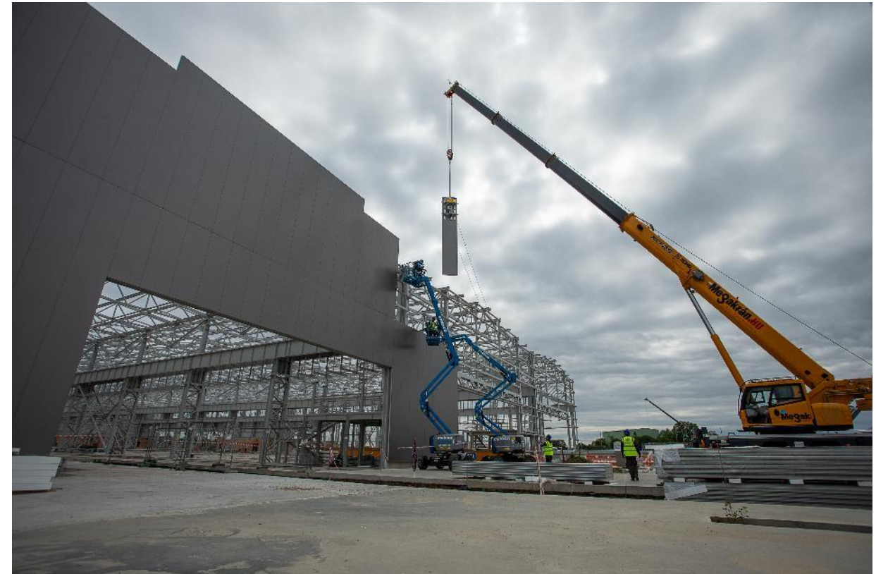
Rebar assembly workshop
