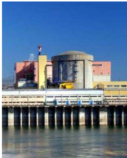
Refurbishment / Life Extension of Unit 1
