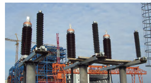
Yulin Dabaochang 110KV Transmission Line Project
