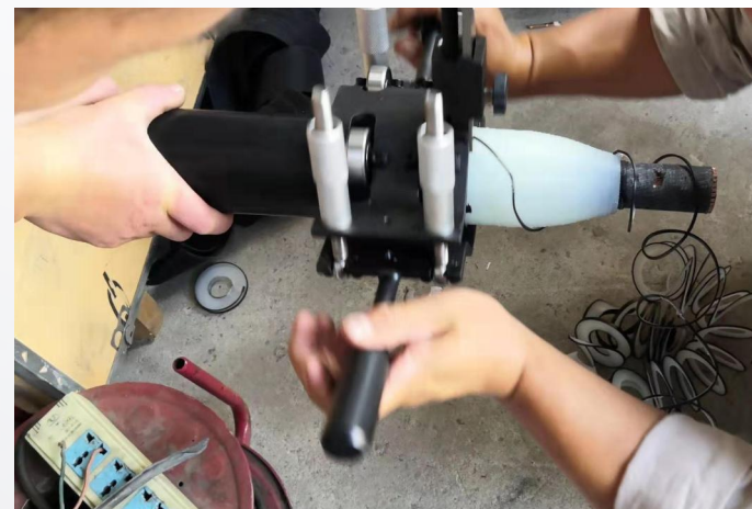
Stripping the cable
