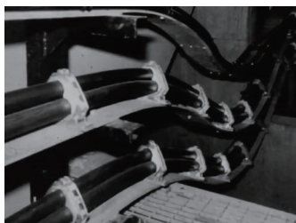
Laying of 132kV Power Cables on the River Lea Bridge in the UK
