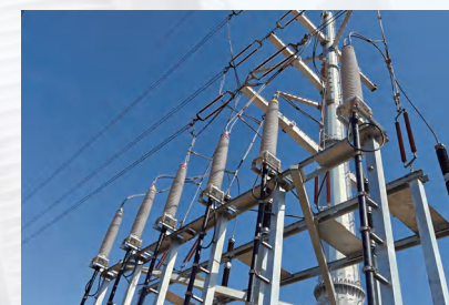
Qinhuai Big Data Center Transmission Project
