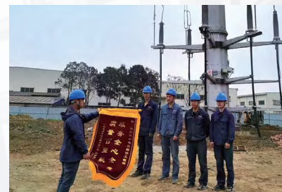
Harbin Bin County Wind Power Project
