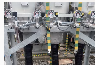
The Fourth Phase New Construction Project of Tongwei Solar in Meishan City
