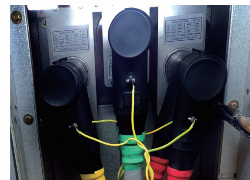
Fabrication of T-type joints for 10kV capacity expansion and transformation of Zhonglian Data 220KV Substation
