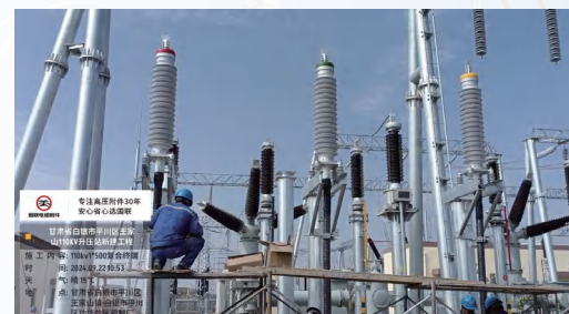
New Construction Project of Wangjiashan 110KV Booster Station Pingchuan District, Baiyin City, Gansu Province
