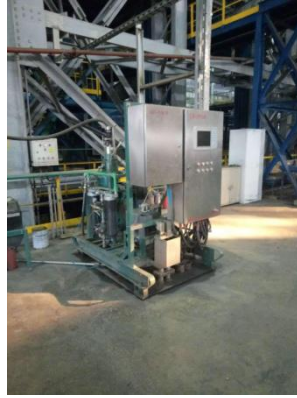
Particle size measurement at cyclone overflow in iron processing plant
